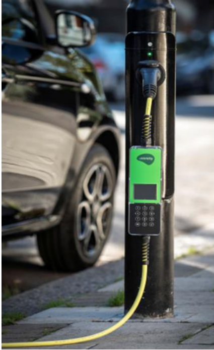
Figure 9 - Lucy Zodion Trojan Midi with 32 A disconnecter
