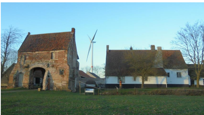
Ecopower's Community Wind Turbine in Eeklo
