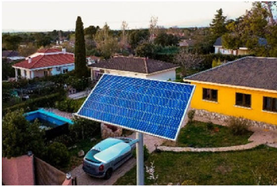
All in two luminaire in residential zone
