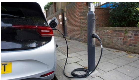
Figure 6 - Simple installation - cable only
