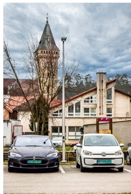
Figure 11 - Installation in Sabinov
