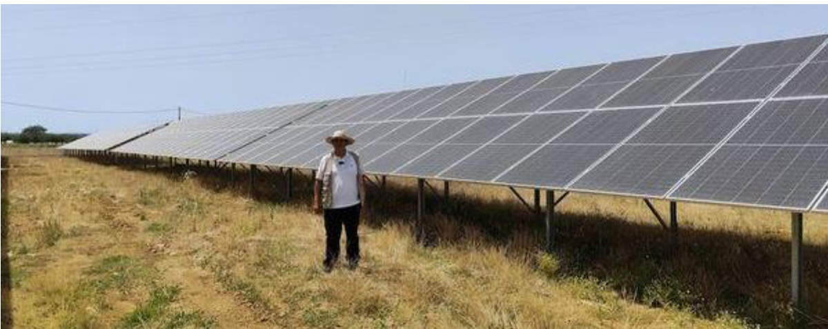
Stages of Construction of the PV Station (Initial land plot, installation of support structures, placement of PV panels, Installation of electrical equipment, PV station with connection to the grid)
